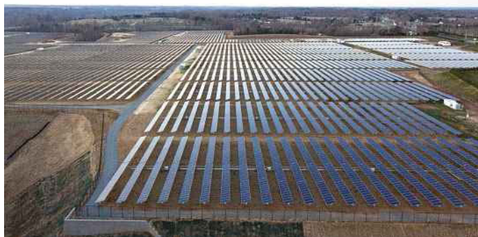
▲ Solar Array at Maiden, North Carolina
